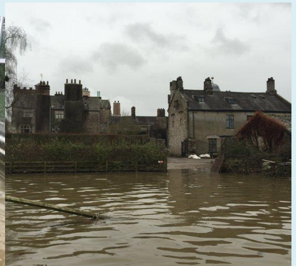
Water enters topiary courtyard
