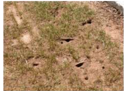
Notice the holes opened by pine voles that extend into the lawn near a new sidewalk where a tree was cut.
